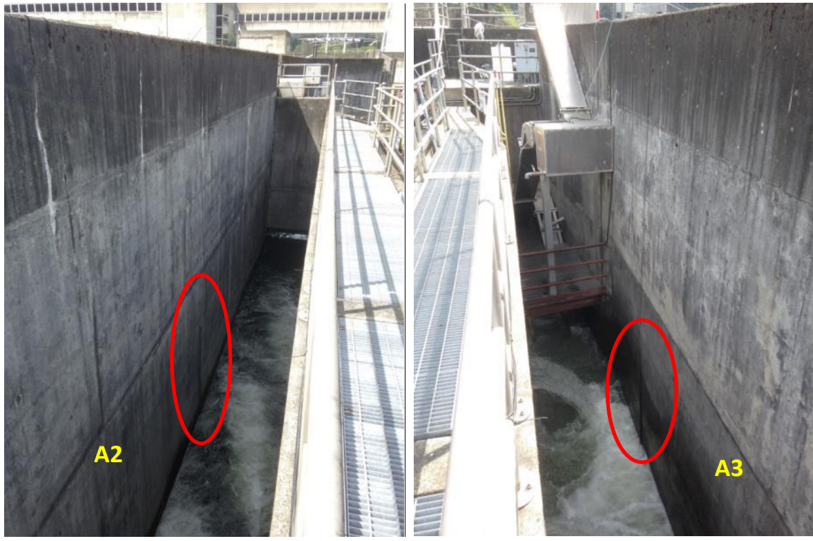
PBO: Washington shore Top-of-Ladder
