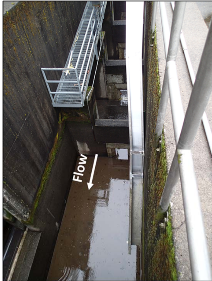
Figure 1. Overhead view of Adult Fish Facility (AFF) lamprey trap in the Washington shore fish ladder at Bonneville Dam.
