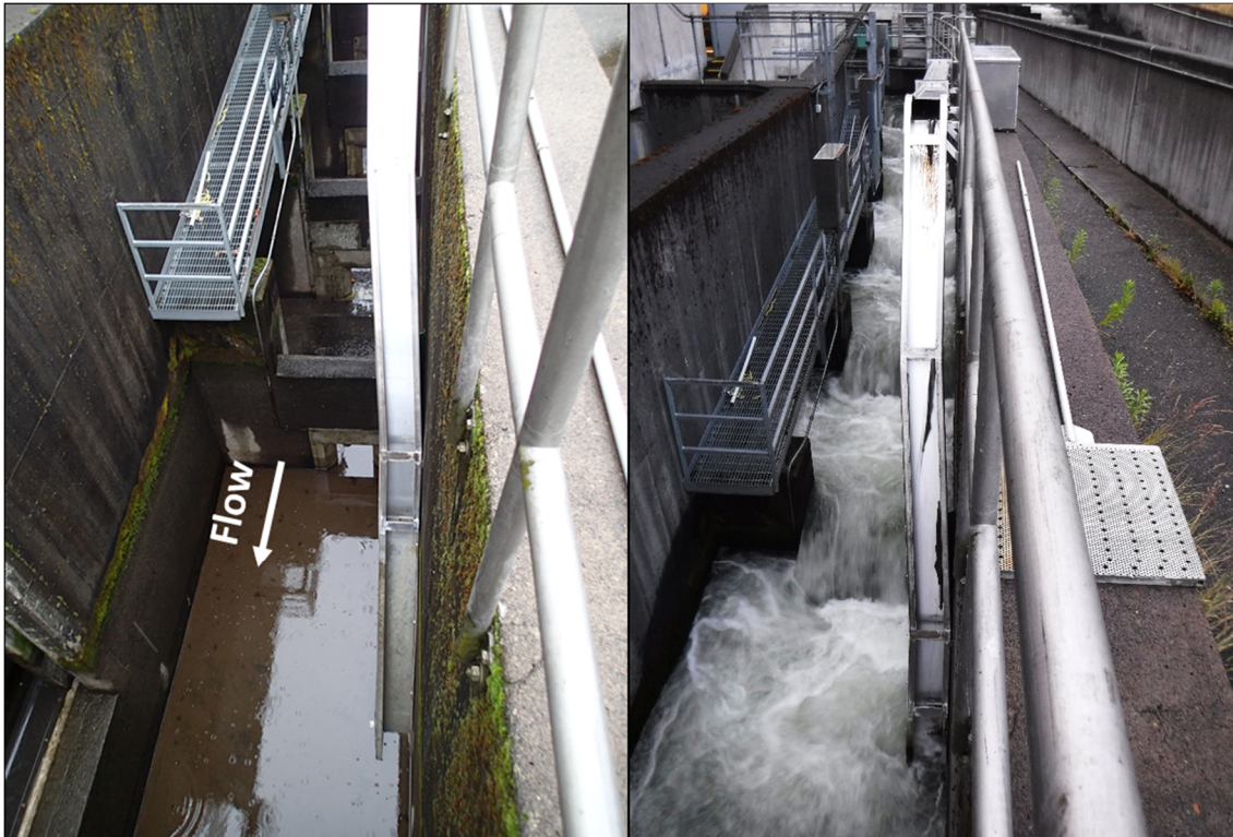
Figure 1. Overhead view of Adult Fish Facility (AFF) lamprey trap dewatered (left) and in operation (right) in the Washington-shore fish ladder at Bonneville Dam.
