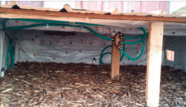
Figure 5. Inside view of a closed-bed biofilter. Photo by Lide Chen.
