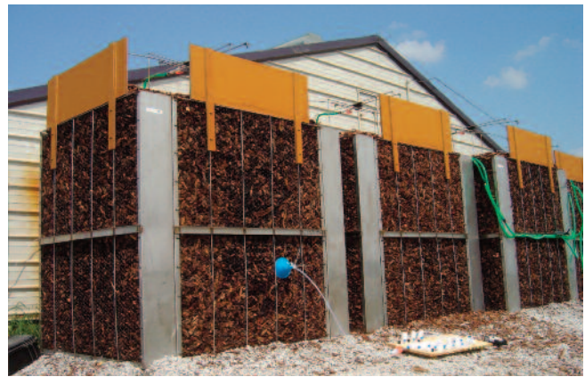
Figure 8. Vertical biofilters. Photo by Lide Chen.
